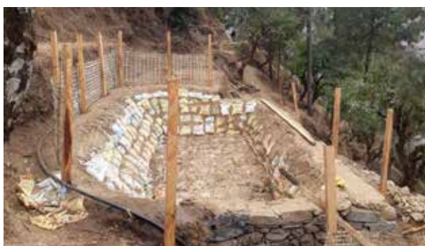
Plastic Pond under construction for rain water harvesting
